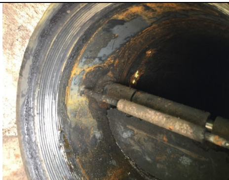
Damaged threads
