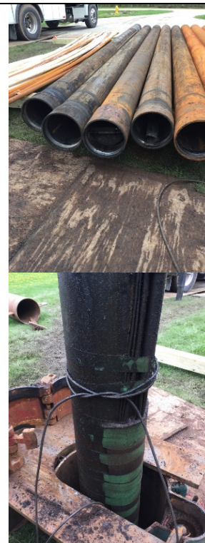
New transducer as well as new transducer conduit should be installed. Old conduit came apart shortly after original install- per client
