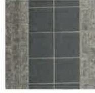
Existing Glazed Blocking Tile
