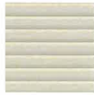
Existing Metal Panels
